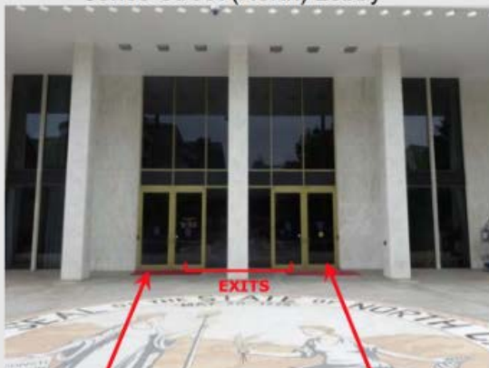
Jones Street (North) Lobby
